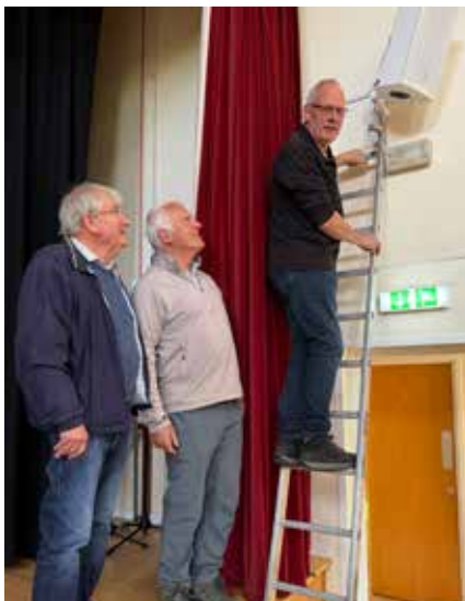
Dennis Booth (left) and Duncan Straughen look on as Andy Callin (Sound Analysts) carries out the installation.
